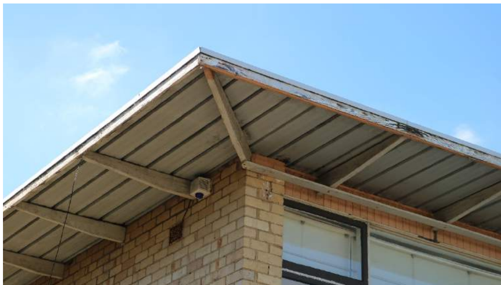
Figure 5. Broad eaves detailing (GJM Heritage, April 2021)
