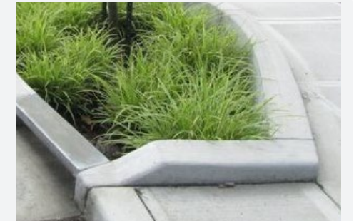
Formed concrete edges
