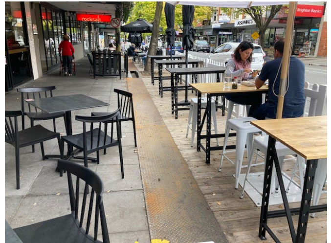
FIGURE 11 – PLATFORM TREATMENT PROVIDED TO CONNECT PARKLET TO KERB
