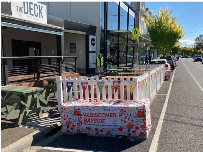
FIGURE 4 – CONCRETE BLOCKS PROVIDED AT EACH END
