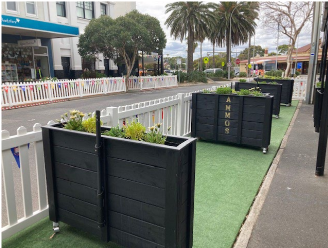
FIGURE 10 – PARKLET PLATFORM SITS FLUSH AGAINST KERB
